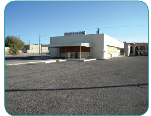
A vacant building on Central Ave. between San Pedro & Louisiana.
